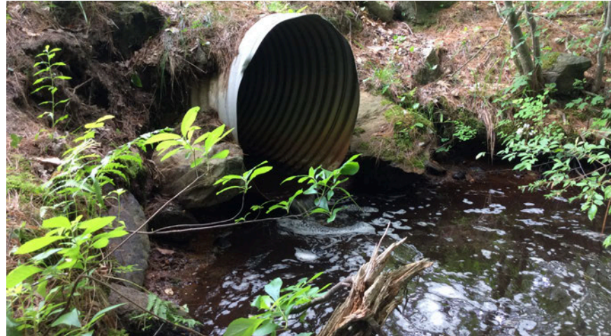
A culvert in Fremont assessed in 2015. Photo via RPC.
