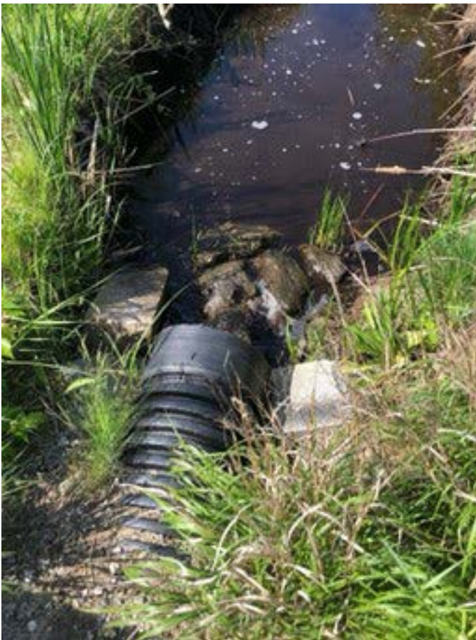
Drainage structures on Parsons Road. Courtesy of Jo Sias (June, 2021).
