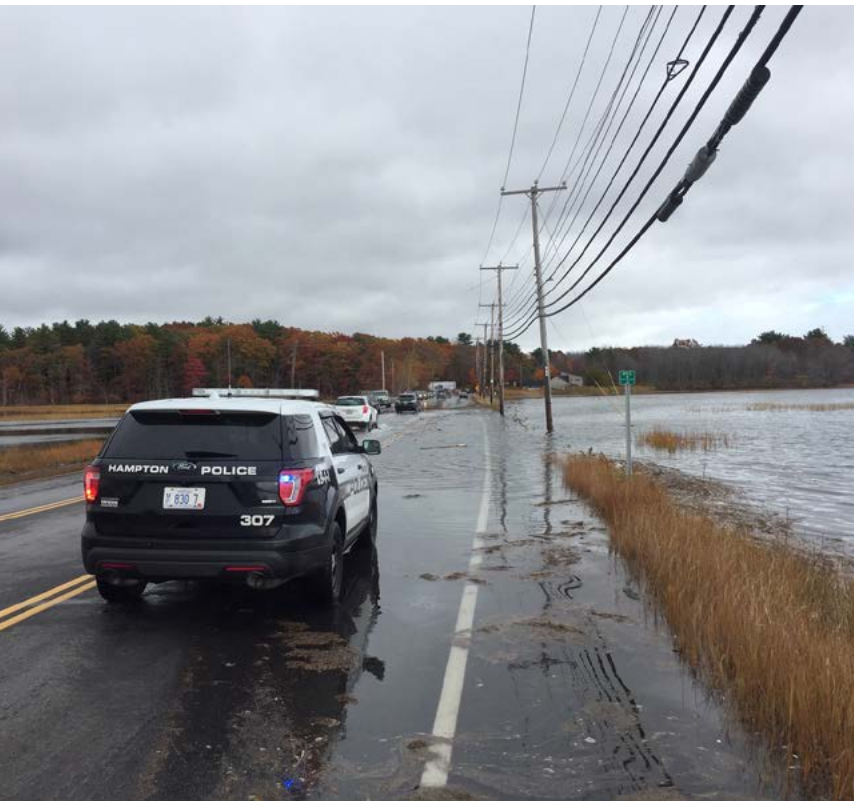
Hampton Police blocking a section of US Route 1 through the Hampton-Seabrook Estuary during high-tide flooding in 2019. Photo courtesy of Scott Bogle.
