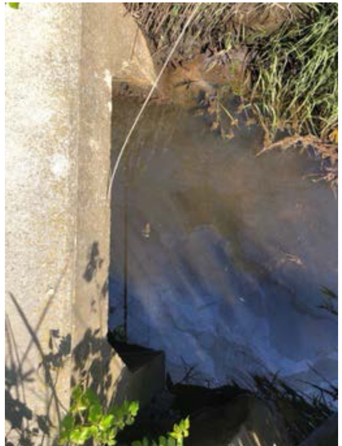
Drainage structures on on Marsh Road. Courtesy of Jo Sias (June, 2021).
