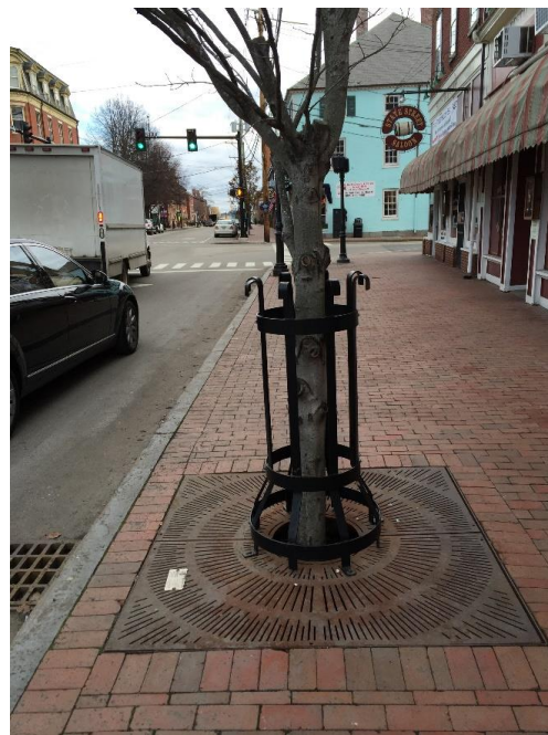
Figure 7: Tree Planter Combined with Catch Basin
