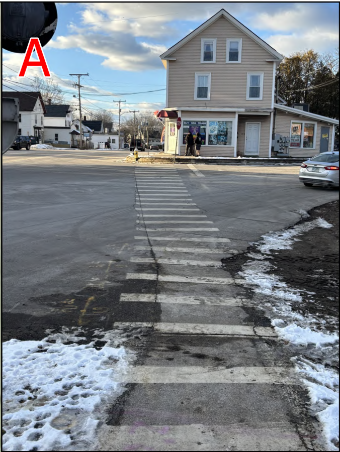
(Left) Looking westward from point A along the 100+' crosswalk, towards Retro World and Pizza Academy. The curb is 12.5" high with no ADA ramp.
