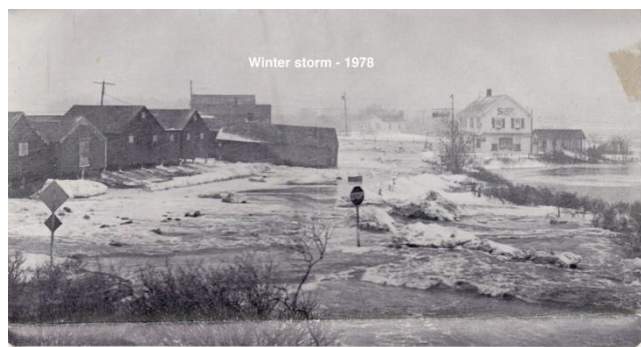
View of Ocean Boulevard in the vicinity of the Fish Houses at the height of the storm on February 7, 1978. Lydia Bottomley's Fish House has just floated onto the State highway, the ocean is flooding into the marsh. P 32. MEB 09 (photo by R.A. Southworth) storm February 7, 1978. Source: North Hampton Historical Society
