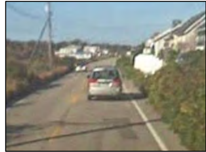
Figure 5.10: Vegetation encroachment onto shoulder south of Jenness
