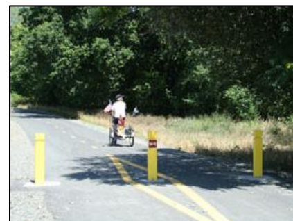
Figure 2. Removable bollard access control at trailhead
