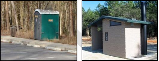
Figure 4. Trailhead restroom facilities, temporary or permanent
