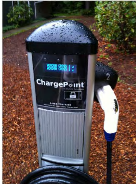
ChargePoint/Coulomb Level 2 Charging Station
