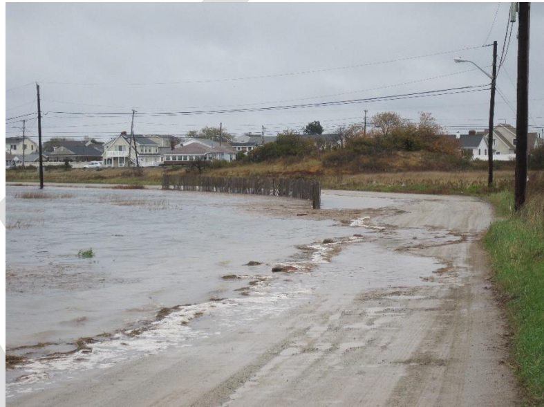
Figure 2. 2013 King Tide flooding at Cross Beach Road.
